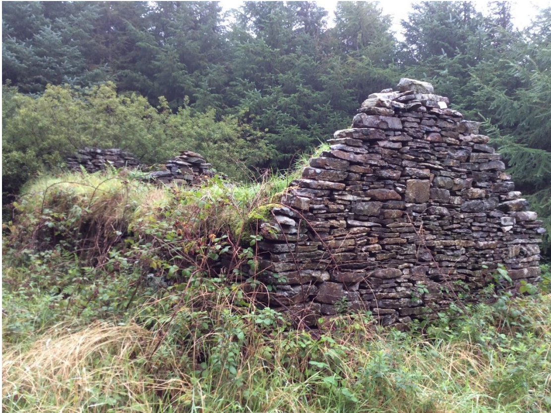
Plate 14-8: CH1 stone structure adjacent to Proposed Grid Connection Site underground cable route.
